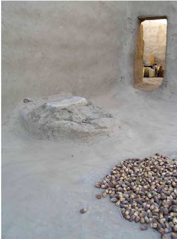
— Mud-plastered walls and floor, with a grinding emplacement and drying dates, within a traditional house on Ernetta Island.
